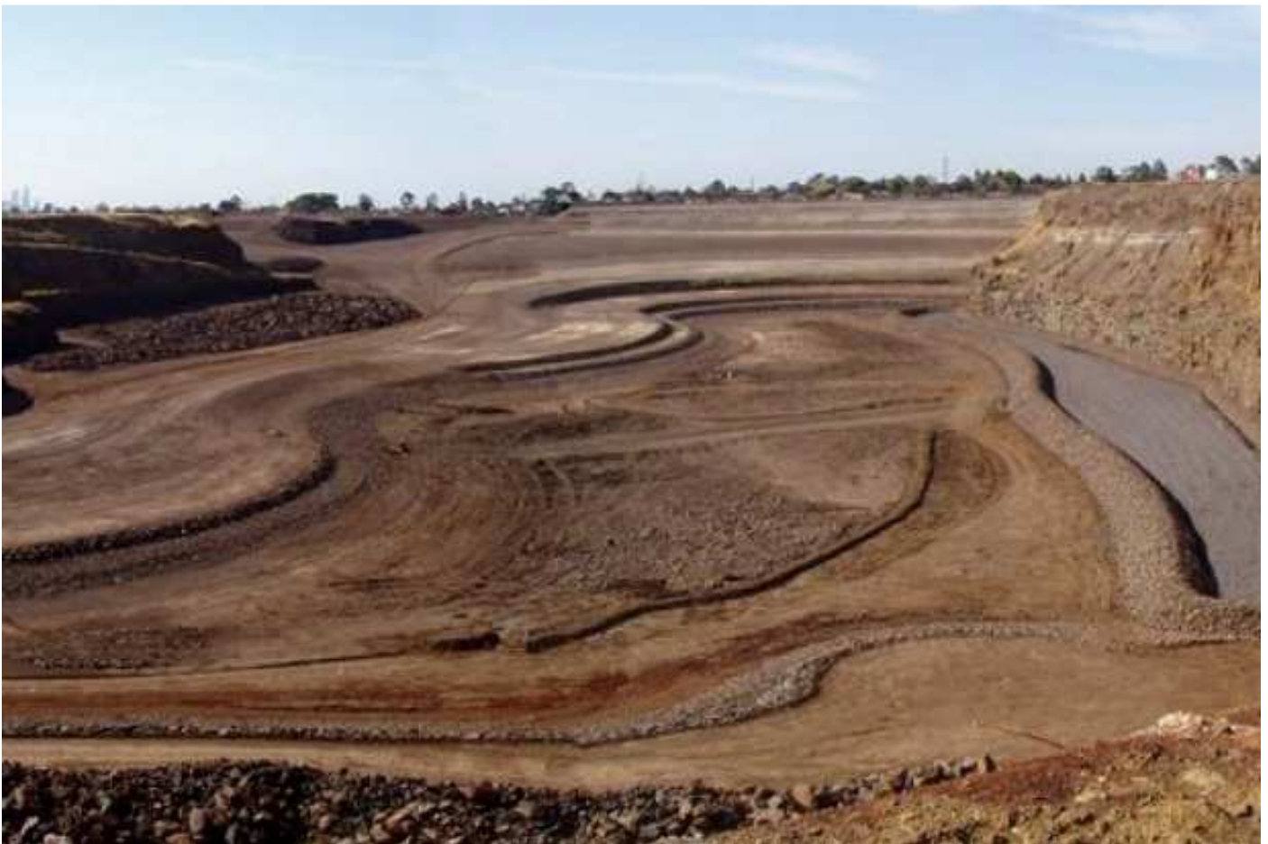
Northern View of Lake Contours after earthworks.
